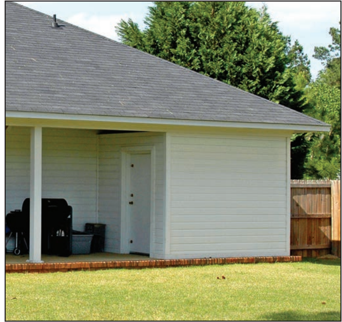
Figure 3-3: An above-ground safe room constructed as an addition to a slab-on-grade home in a way that matches the aesthetics of the home (outside Tuscaloosa, AL, 2011)
